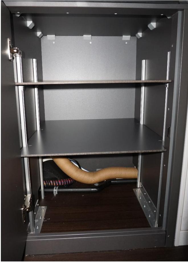
Figure 7. Positioning of aluminium tracks and shelves
