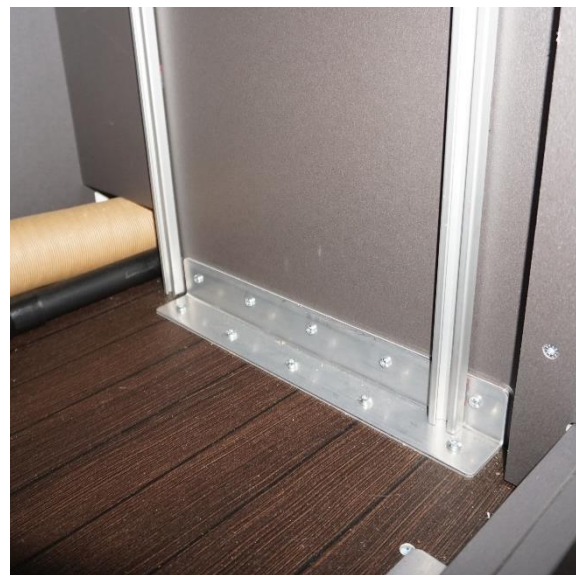
Figure 6. Positioning of aluminium track (B) right hand side.
